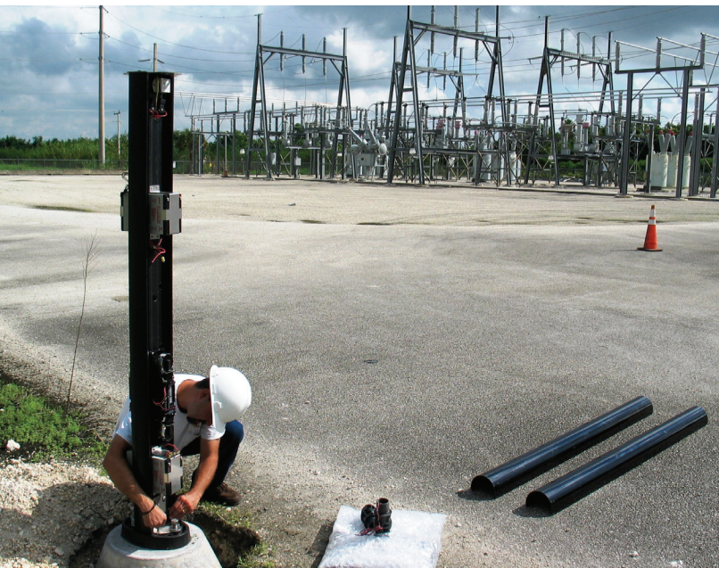
City of Homestead Substation Installation
